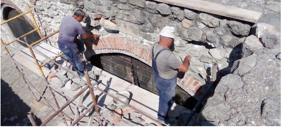
Figure 3: Restoration works on the Public observatory exterior.
